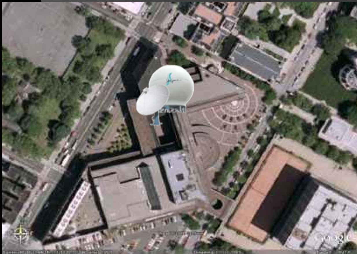
NAC building roof
