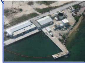
KEY WEST Marine Corrosion
